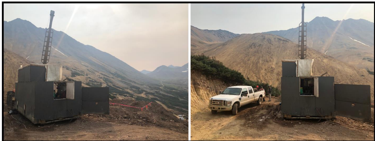
Figure 4. Drill rig during drilling of hole BRG23-245.
